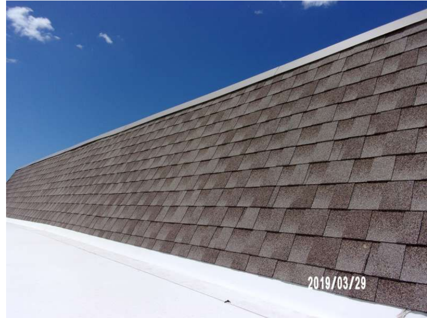
Architectural/Dimensional Shingle Roof Coverage
