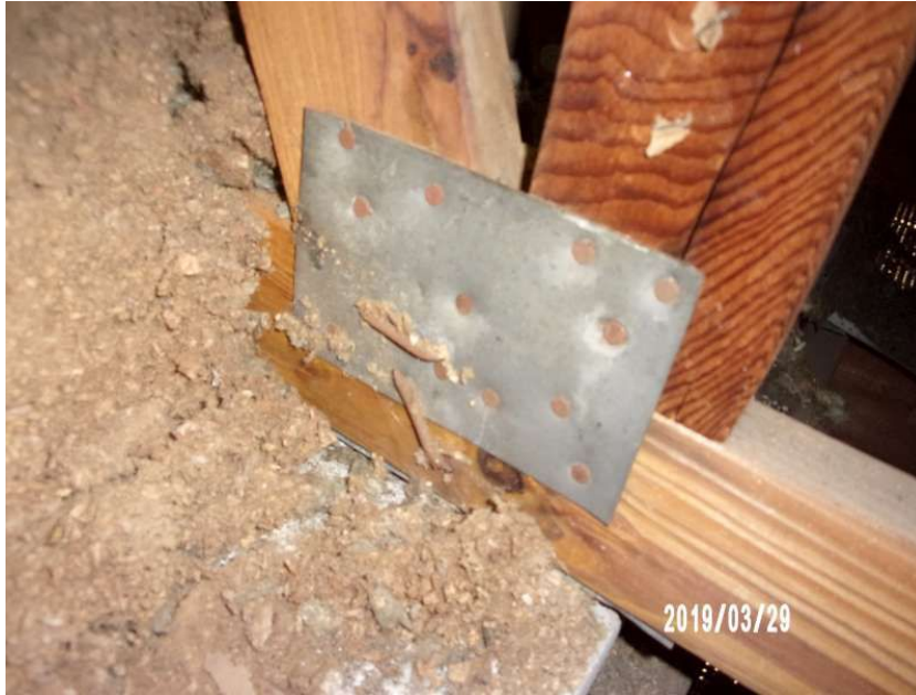
Metal Connector with 2 Nails on the Front Side & 0 Nails on the Opposing Side
