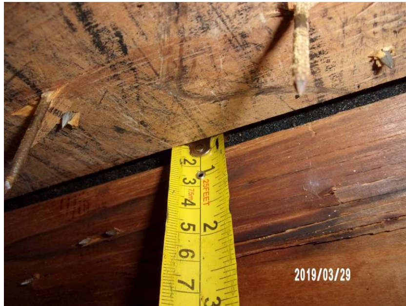
1/2" Deck Thickness Confirmed
