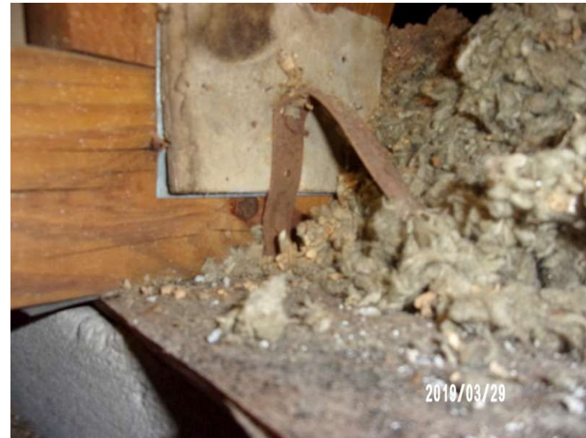
Metal Connector with 2 Nails on the Front Side & 0 Nails on the Opposing Side
