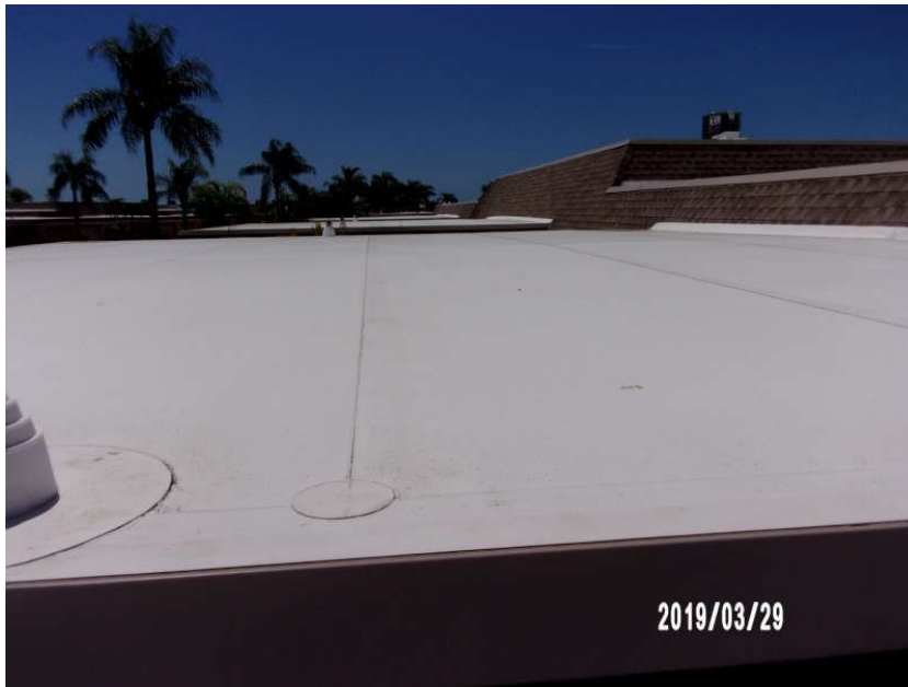
Membrane Roof Covering
