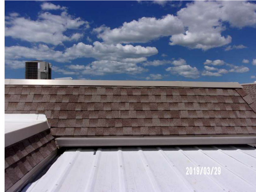
Architectural/Dimensional Shingle Roof Covering
